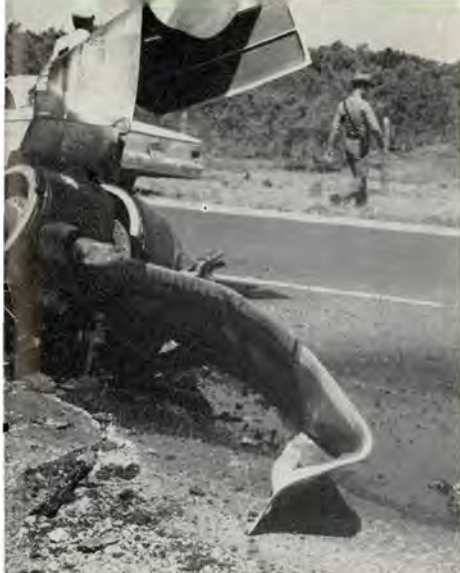
A spectacular example of materiel failure. This engine tore itself from the wing as the airplane flew overhead.
